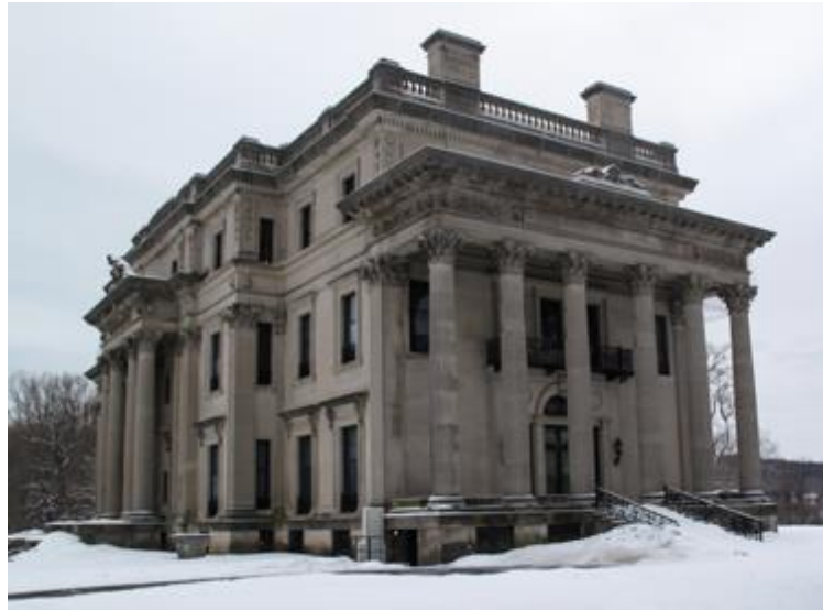
Fig. 12. Conspicuous Noncombustion: Vanderbilt Mansion, Hyde Park (McKim, Mead and White, late 1890s). Its steel and concrete skeleton and stone facing were costly yet powerful signifiers of the Vanderbilts' invulnerability to fire. (Patrick Stahl)
