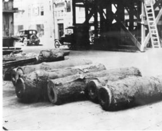
Fig. 3. Excavated nineteenth-century wooden water mains. (Philadelphia Water Department Historical Collection)
