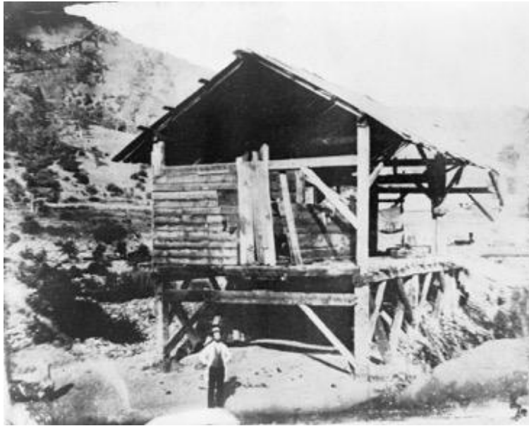
Fig. 5. Sutter's Mill, with carpenter James Marshall standing outside it, exemplifies the hasty wooden construction favoured by nineteenth-century settlers. (Library of Congress)
