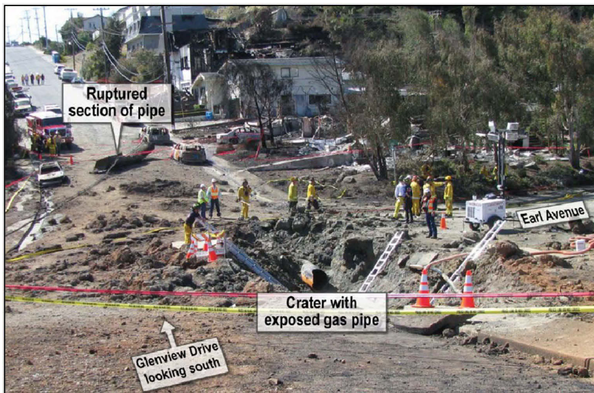
FIGURE 4-5 Site of the San Bruno gas transmission pipeline rupture. SOURCE: NTSB. 2011. Pacific Gas and Electric Company Natural Gas Transmission Pipeline Rupture and Fire, San Bruno, California, September 9, 2010. NTSB/ PAR-11/01. Washington, DC.
